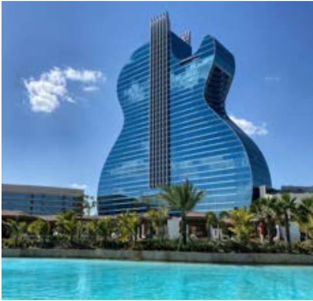
Seminole Hard Rock Hollywood Hotel & Casino Hollywood, FL
