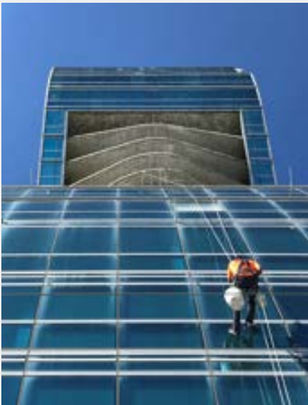
Credits: Top Pixaby\ Bottom left : Bonded Lightning Protection Solutions
